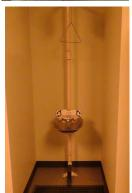
**Safety Showers Function:** For chemical decontamination on a person or their clothing. **Use:** Pull lever for body wash. **Location:** E152 near the double door exit and Chase and Mechanic room.
